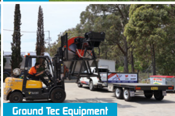
Ground Tec Equipment
